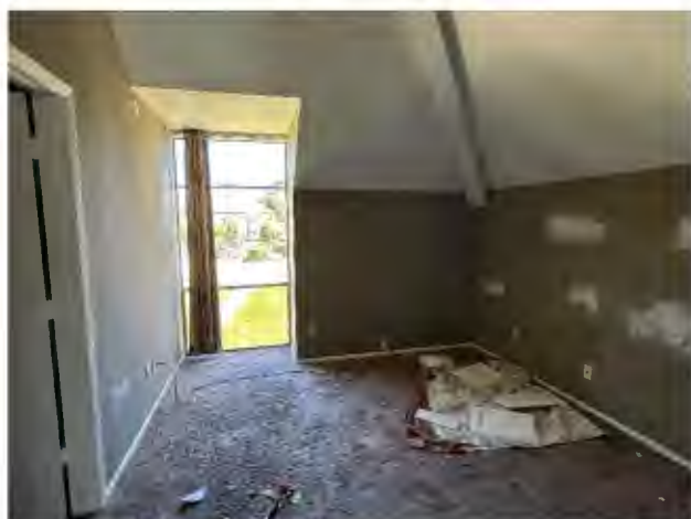
Bedroom (Under Renovation)
