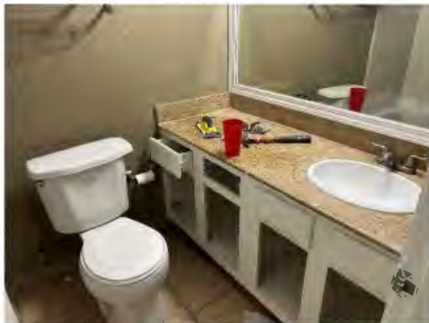
Bathroom (Under Renovation)
