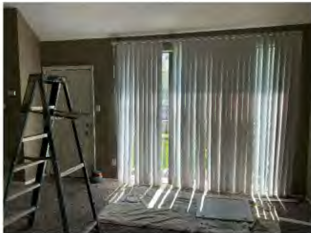
Living Room (Under Renovation)
