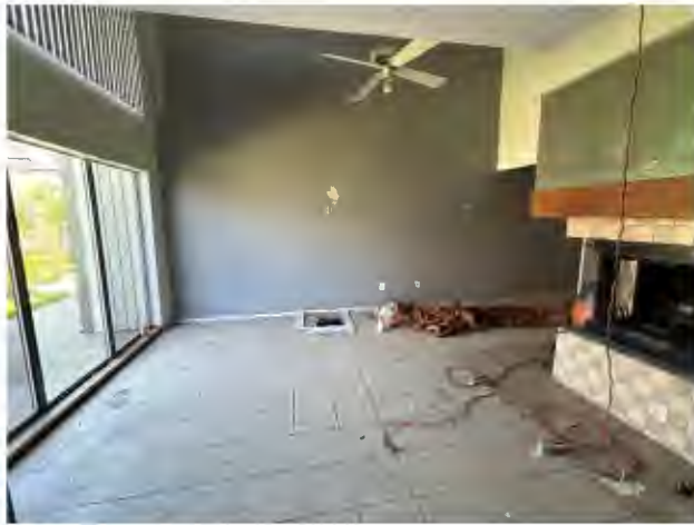
Two-Story Unit (Under Renovation)
