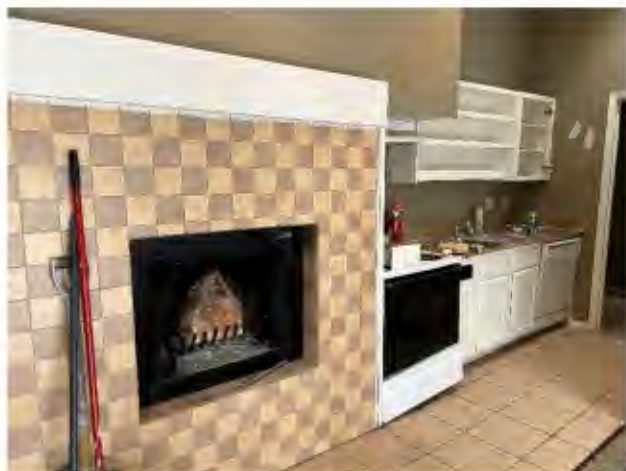
Kitchen (Under Renovation)
