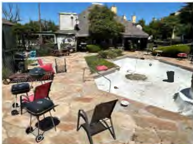
Pool Area (Under Renovation)
